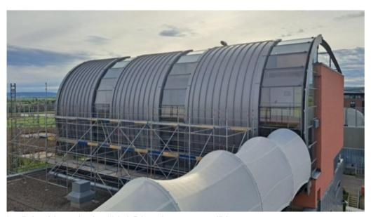
Installation of the new facade at Melexis Erfurt to improve energy efficiency
